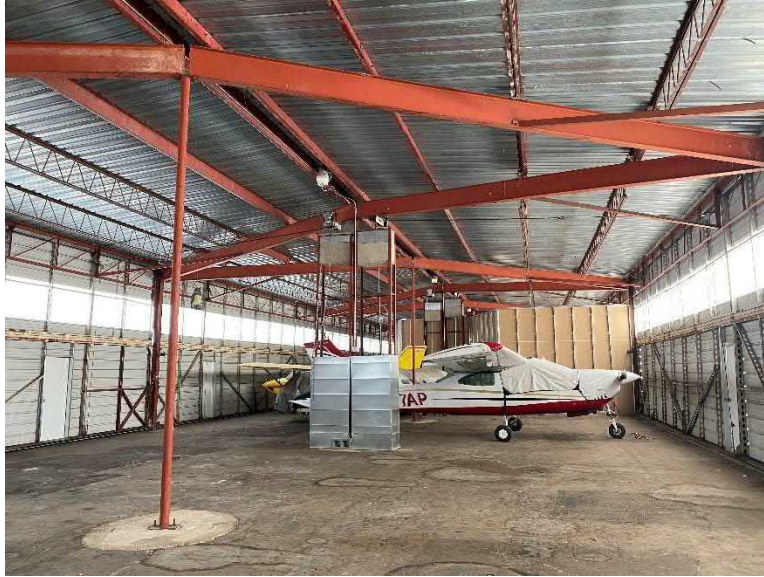
Figure 7. East T-Hangar Interior and Manual Hangar Door Operation
