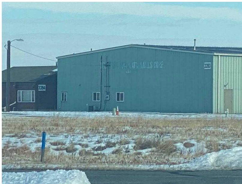
Figure 10. Typical Box Hangar and Office Space
