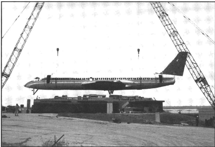
It took over 2 1/2 days to get the Convair off the top of the building and another few days to chew it up and truck it out. Photo taken Friday November 15, 1996 (photo by Bill Diesch).
