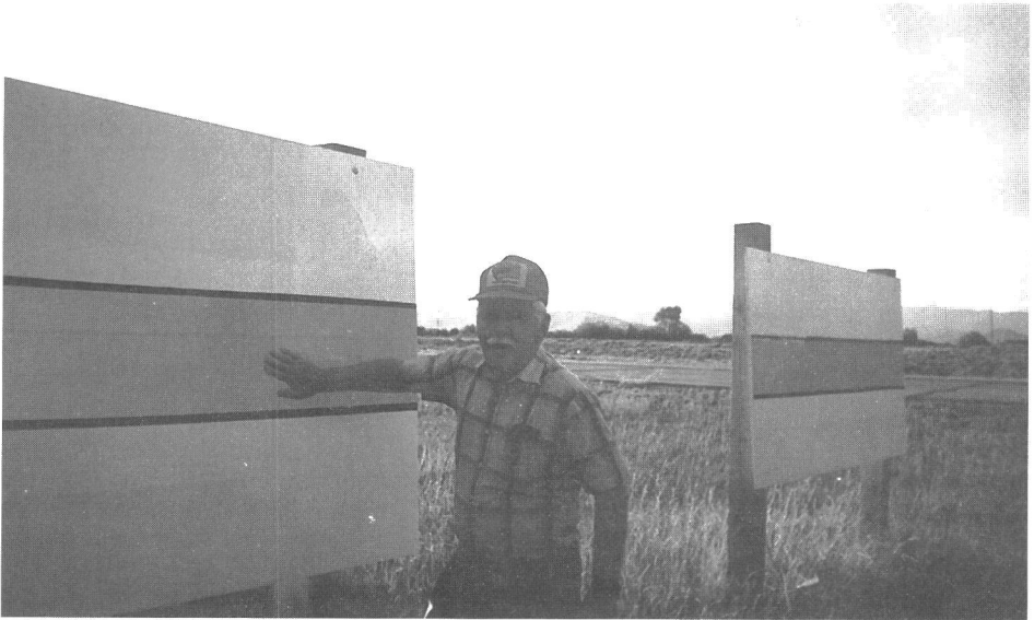
CPAer, Bob Doubek, applies orange reflecting tape to a CIA-VASI panel at GNB.
