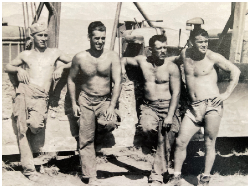
Marion A. Harrison, second from left with three of his Army buddies, in front of their bulldozers, Los Alamos, New Mexico, 1944-1945
