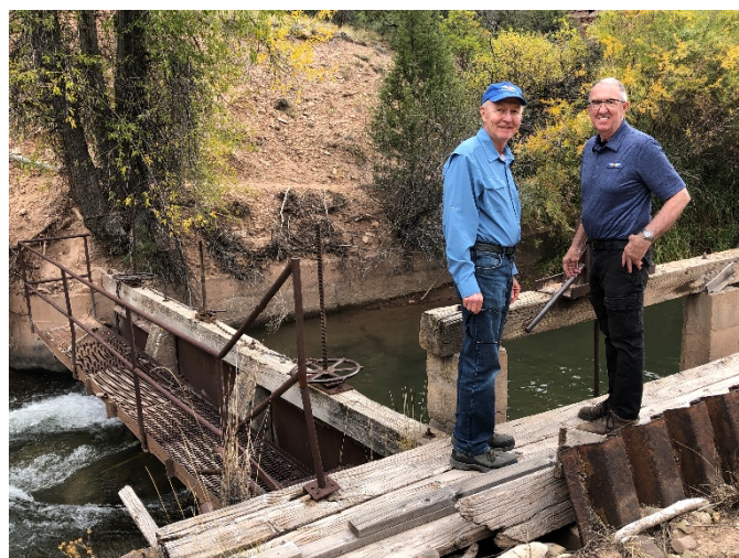
Bill Gust and John Head inspect the headgate of the 20-mile-long ditch. This is where it starts, taking water from the San Miguel River downhill to supply the small towns below.
